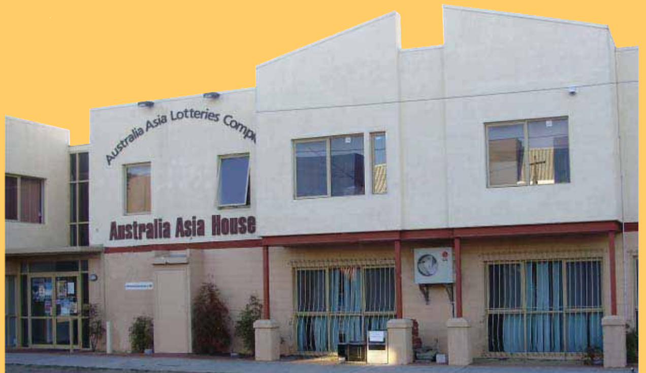
AUSTRALIA ASIA LOTTERIES COMPLEX
